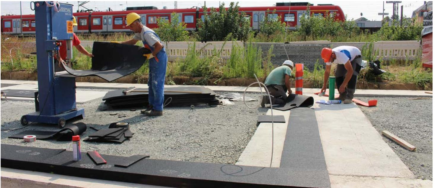
The housing precinct "Quellenpark" has successfully managed these obstacles. A 300-meter-long building complex has been built parallel to the railway track in a distance of just 14 m. Thanks to an elastic decoupling of the building's strip foundations this development is being protected against ground-borne vibration and secondary air-borne sound.
