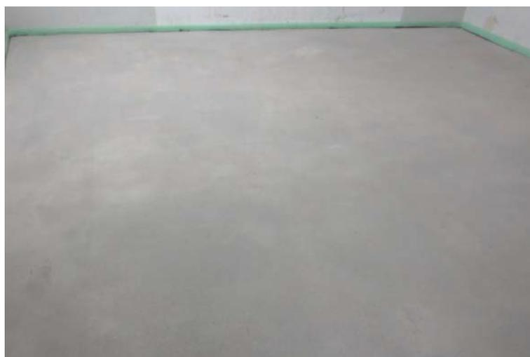
**Picture A 2.3:** completed floating floor screed (situation for test)
