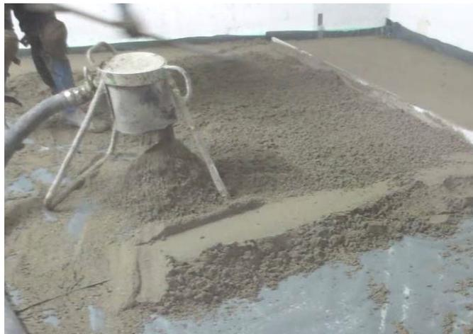
**Picture A 2.2:** mounting situation with floating floor cement screed
