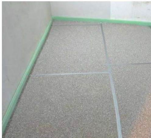
**Picture A 2.1:** mounting situation with impact sound insulating material and edge insulation strips
