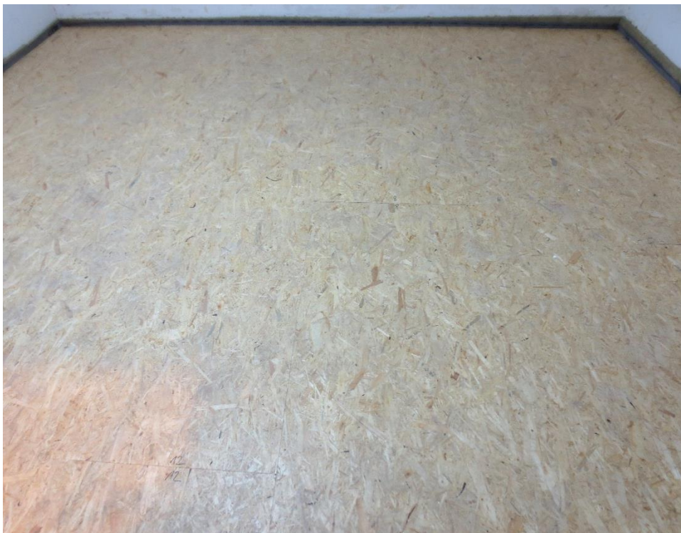
Figure A 2.5: dry screed (situation of test)
